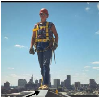
Clearance for lanyards designed for severe free fall can add 6 inches to clearance distance
